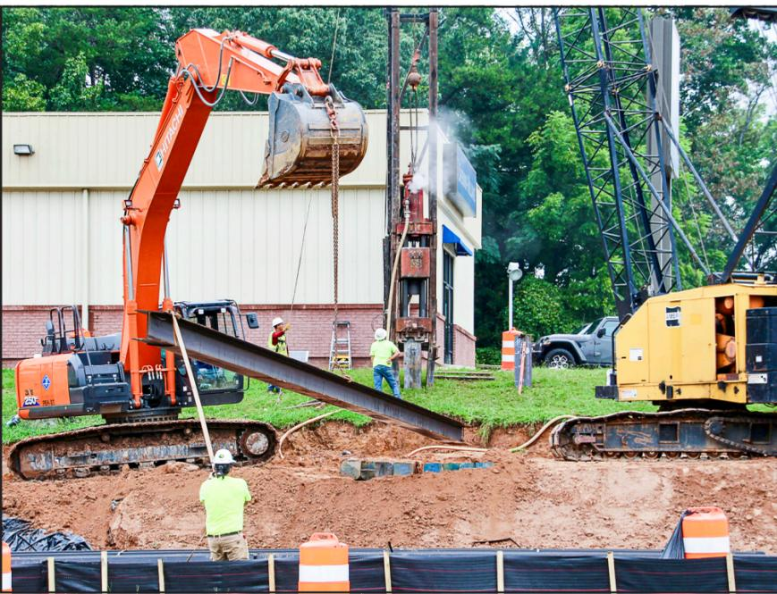
Workers maneuvering a massive steel beam into place before loading it into a pile driver to shore up dirt near the Murphy Highway/515 sinkhole. Photo by Shawn Jarrard
